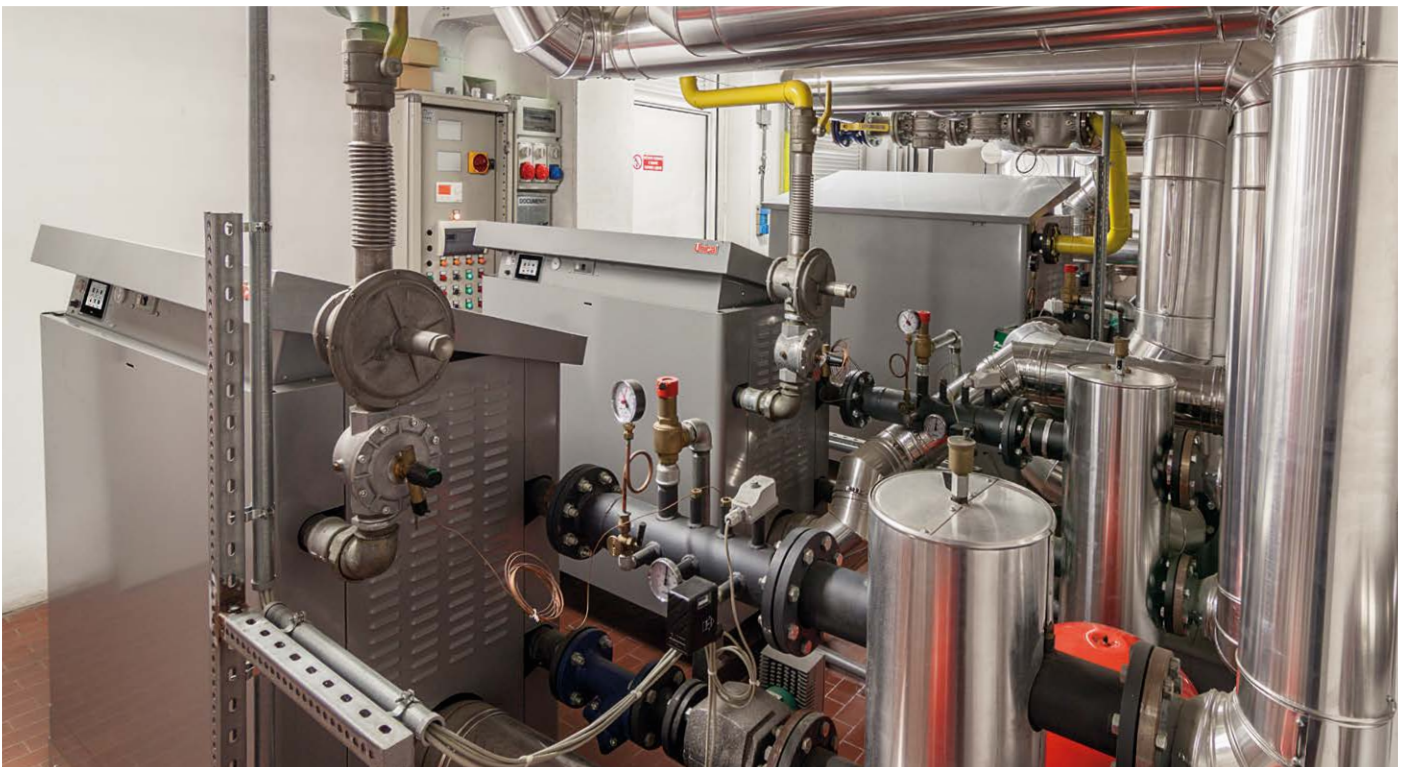
INSTALLATION IN BOILER HOUSE
